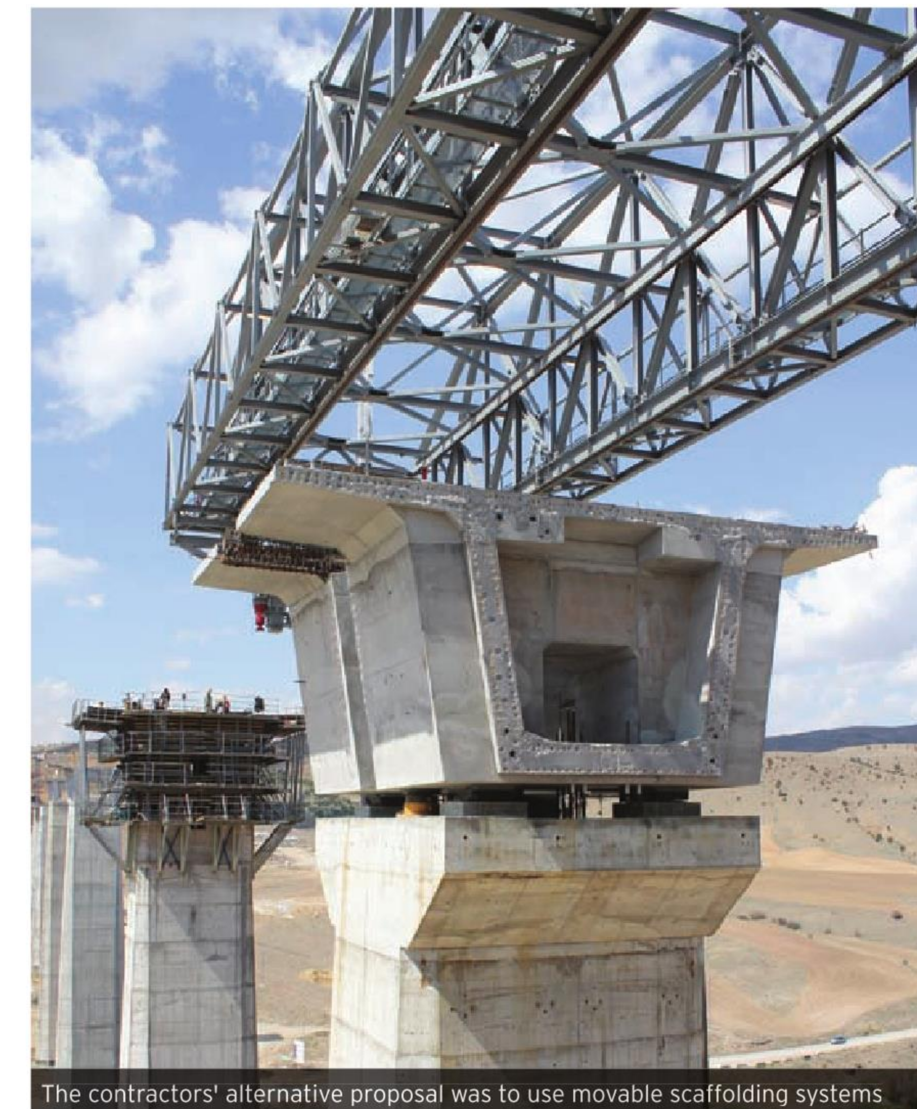
The contractors' alternative proposal was to use movable scaffolding systems
